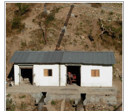
Fig. 7. EP's multi-purpose electromechanical MHP system.
